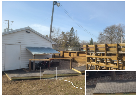
Above: The walkway after Ziegler rebuilt it.
